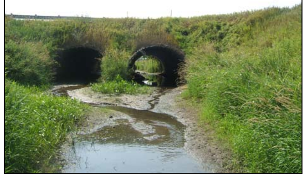
Figure C: Remy-Chandler Drain upstream of State Road.
