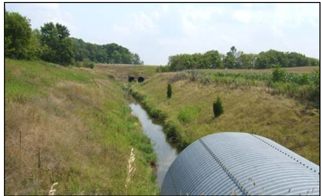
Figure D: Remy-Chandler Drain upstream of Wood Road
